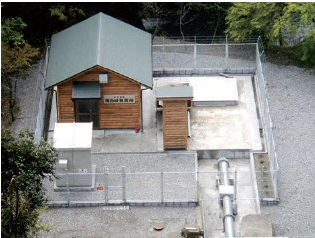
■ 図1 発電所の全景 Fig.1 Whole View of Power Station
