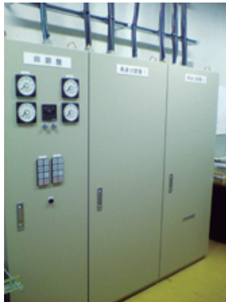
Fig.2 High-speed Change-over Panel
