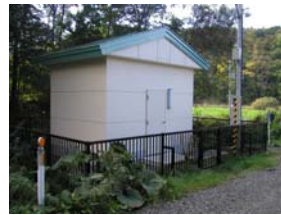
図3 量水器室 Fig.3 Measurement room
