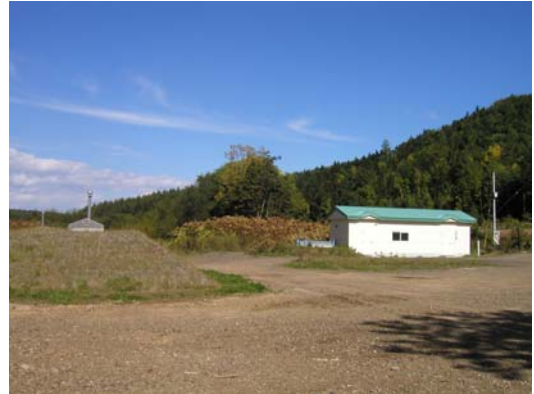
図2 取水場・送水ポンプ場 Fig.2 Nikura water supply plant
