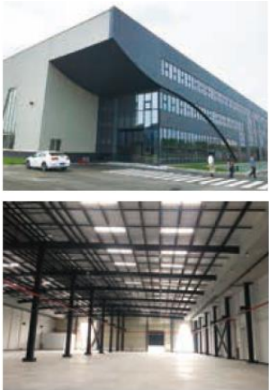
Exterior and interior of Chinalco Toyo
