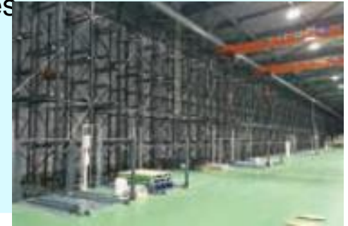
Utilizing TDS (Automatic warehouse system).
