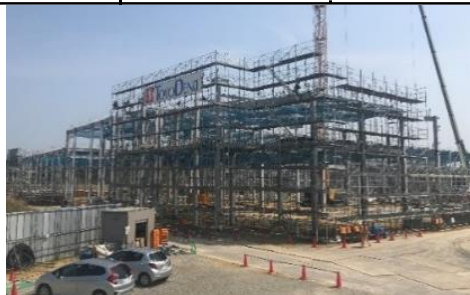
Current status of construction of Shiga Ryuo Works at the end of June
