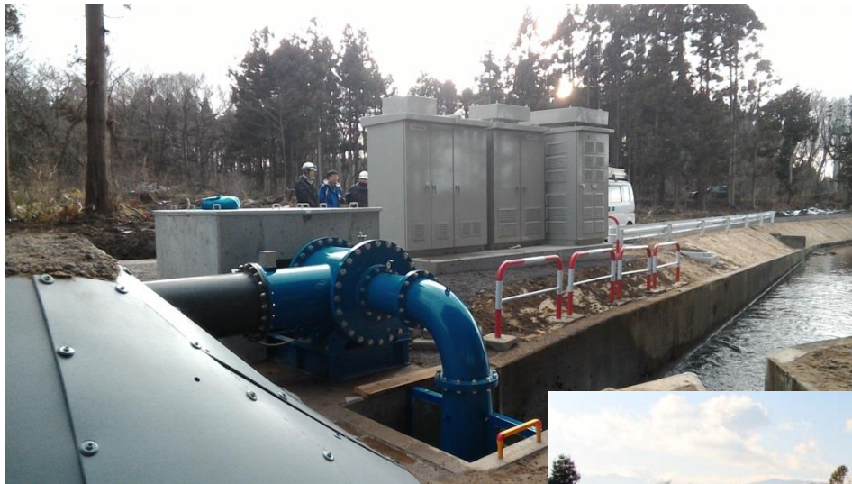
Pumped small hydroelectric power generator in Nikaho City, Akita Prefecture
