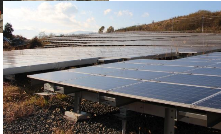
Yonekurayama Solar Power Plant in Kofu City, Yamanashi Prefecture
