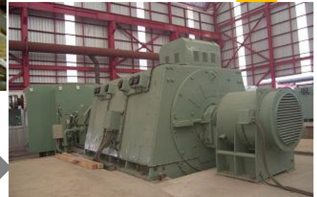
Biomass power generation system
