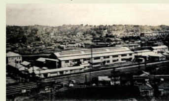
Yokohama factory at the start of operations (Hodogaya-ku, Yokohama)
