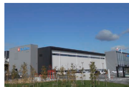
Shiga Ryuo Plant
