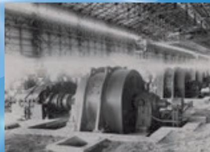
Electrical equipment for medium-sized shape steel rolling equipment (1961)
