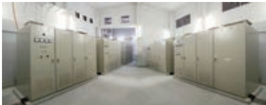
A railway power storage solution, E 3 Solution System (Delivered to TOBU RAILWAY CO., LTD.)
