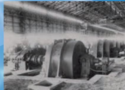
Electrical equipment for medium-sized shape steel rolling equipment (1961)
