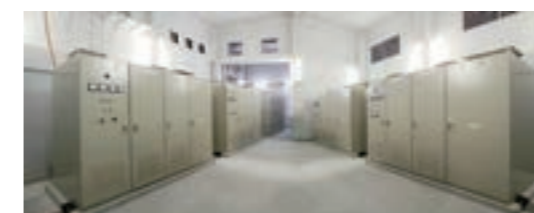
A railway power storage solution, E 3 Solution System (Delivered to TOBU RAILWAY CO., LTD.)
