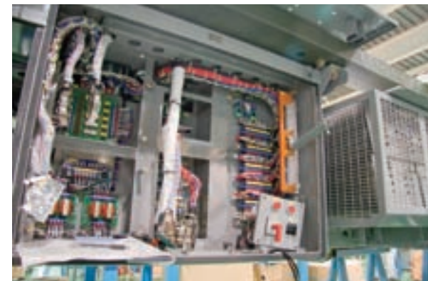
A VVVF Inverter
