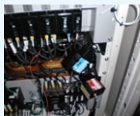
Installation of battery-free sensors
